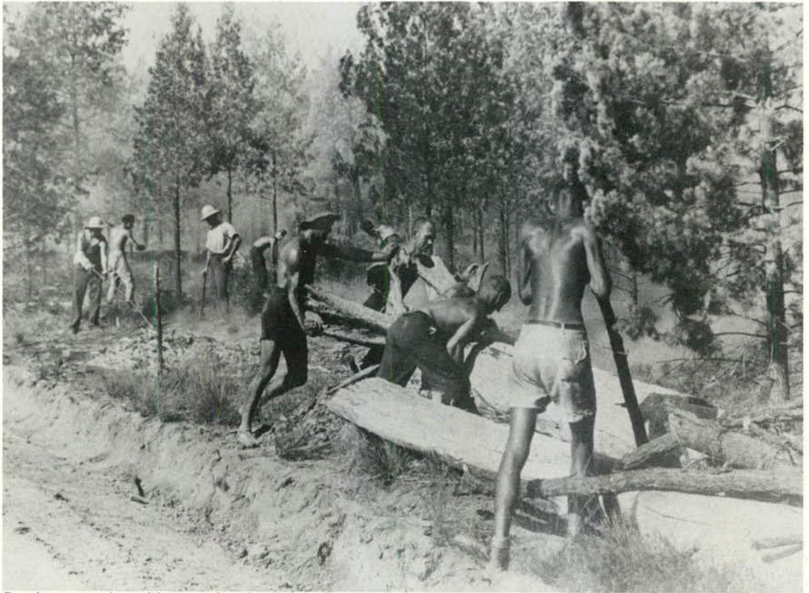
Road construction with unemployed relief workers, 1930.
